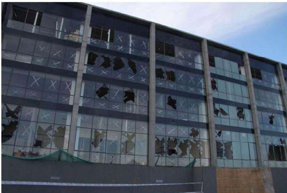
Figure 6.3.1.4-3 Glazing damage was observed in many residential and commercial buildings and hospitals throughout central Chile following the 2010 magnitude-8.8 Chile Earthquake (Photo courtesy of Eduardo Miranda, Stanford University).
